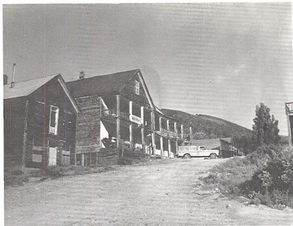
FIGURE 2-29. Idaho Hotel (Block 4, Lots 78 - 80). Present use is a dwelling and cafe.
